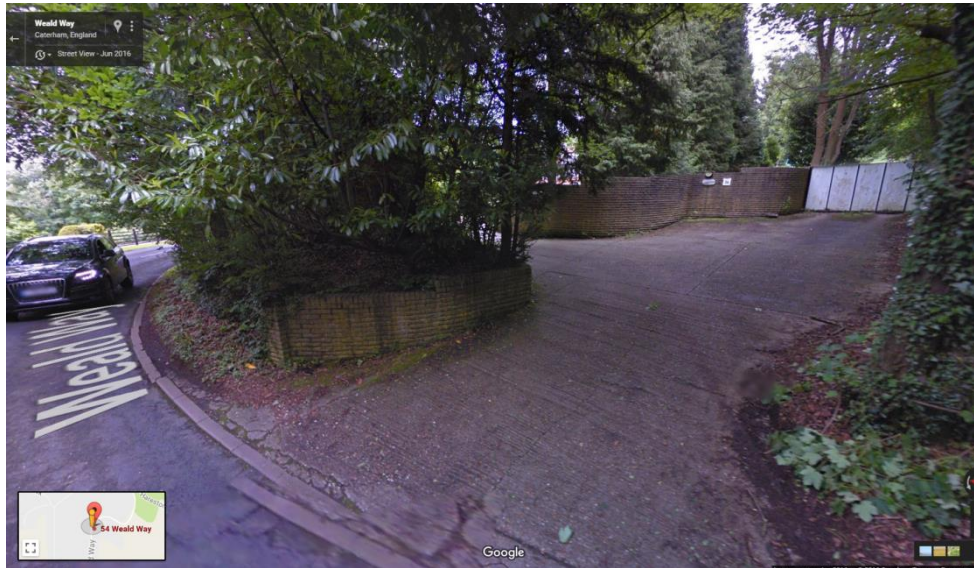
Driveway access to house
